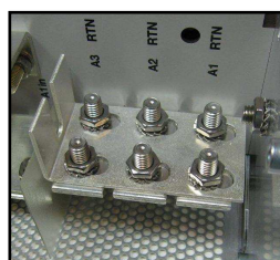
Fig. 8a – Common Return, ungrounded (A Side – flange pointing up)
