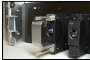
Fig. 13a – Removal tool attached to breaker
