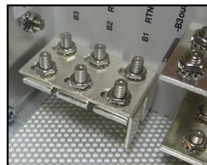
Fig. 8b – Common Return, ungrounded (B Side – flange pointing down)
